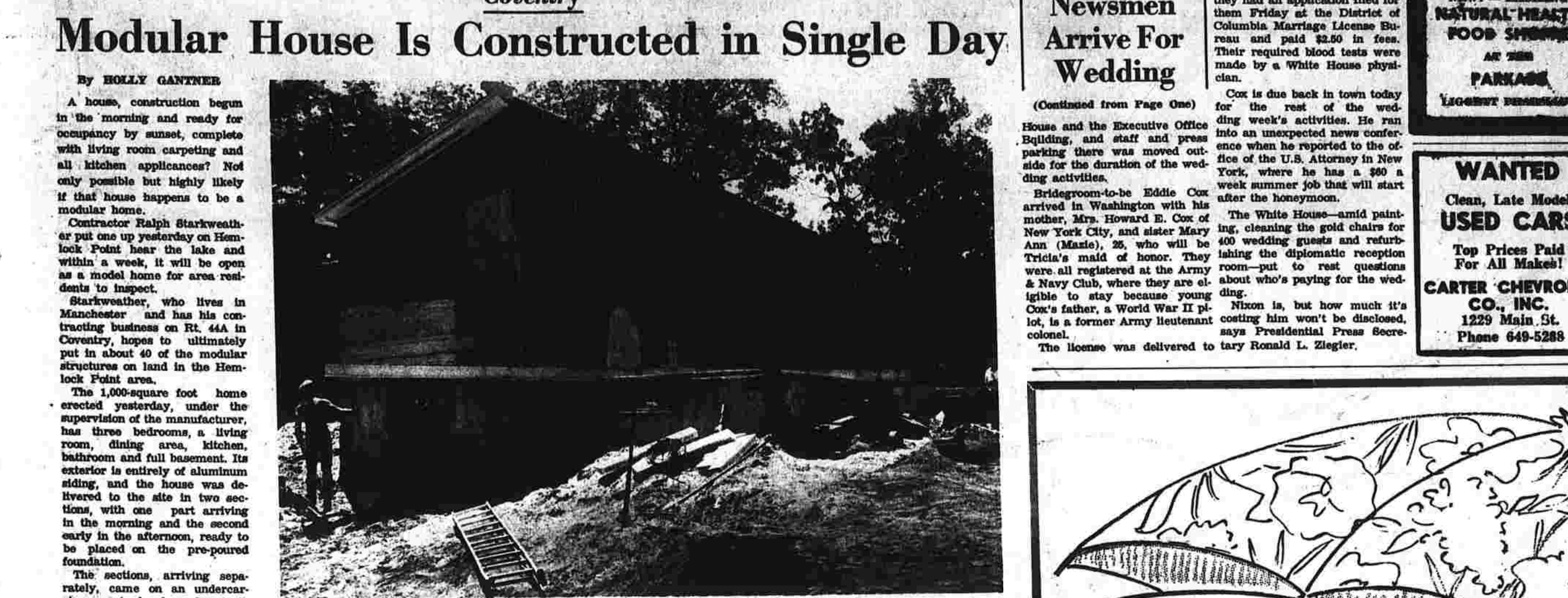
Workman inspects alignment with foundation on first half of modular house. (Herald photo by Leggett)
