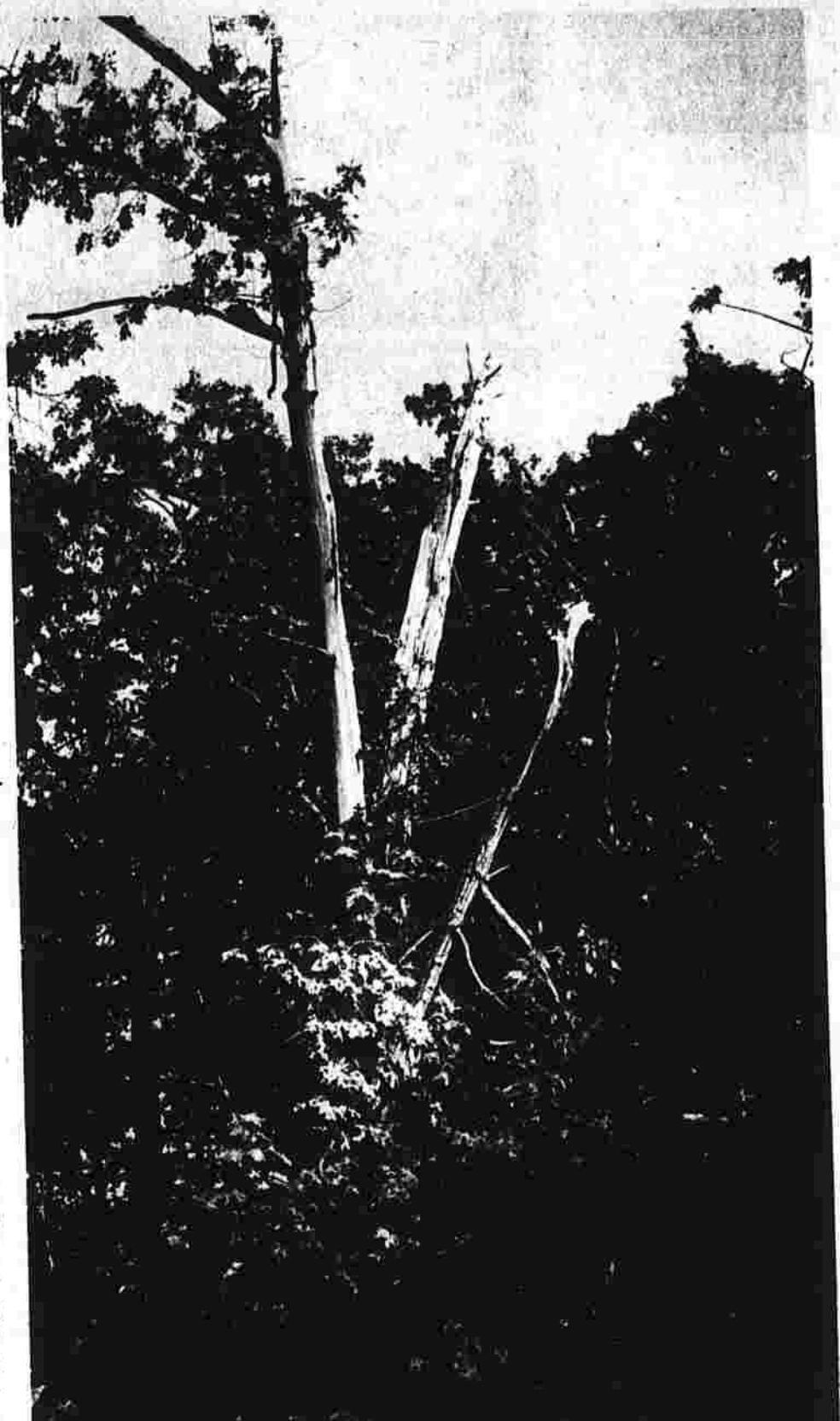
Split by lightning at the height of last night's electrical storm, this 100-foot oak, in the yard of Mr. and Mrs. Allan Cose of 114 Vernon St., was reduced to splinters and strewn over a wide area. Lightning also knocked off the telephone box and blew fuses throughout the house, Cose said. He is principal at Bannet Junior High School. (Herald photo by Eucelvicus)
